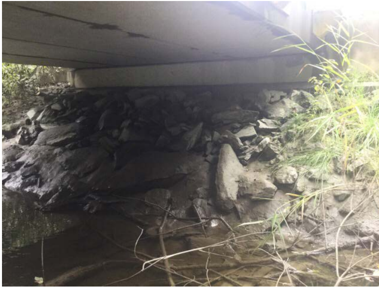
Right Bank Abutment when facing downstream
