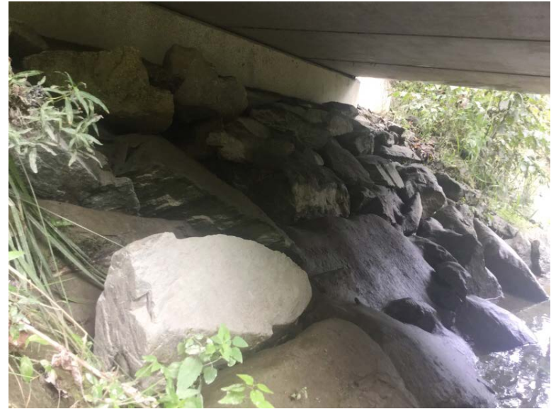
Left Bank Abutment when facing downstream
